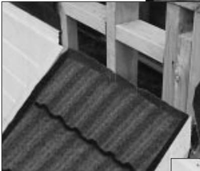
Then add flashing, or if flashing is already there, slide tile up under flashing and secure.
