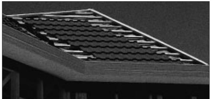
Where laying tiles around skylights, or anywhere where a trim won't be put over it, use a thin strip of flashing to cover up the cut and bent edge of tiles.
