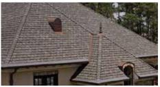
Bitumen, or asphalt, shingles are made from paper and fibreglass, coated with bitumen and asphalt, and ceramic granules. Expensive to install as they need a plywood deck & each tile needs fixing individually. Susceptible to fire and heavy rainfall causes permanent damage. UV damage means frequent replacement
